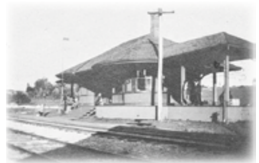
N. Newport station Credit: Larry Cote
